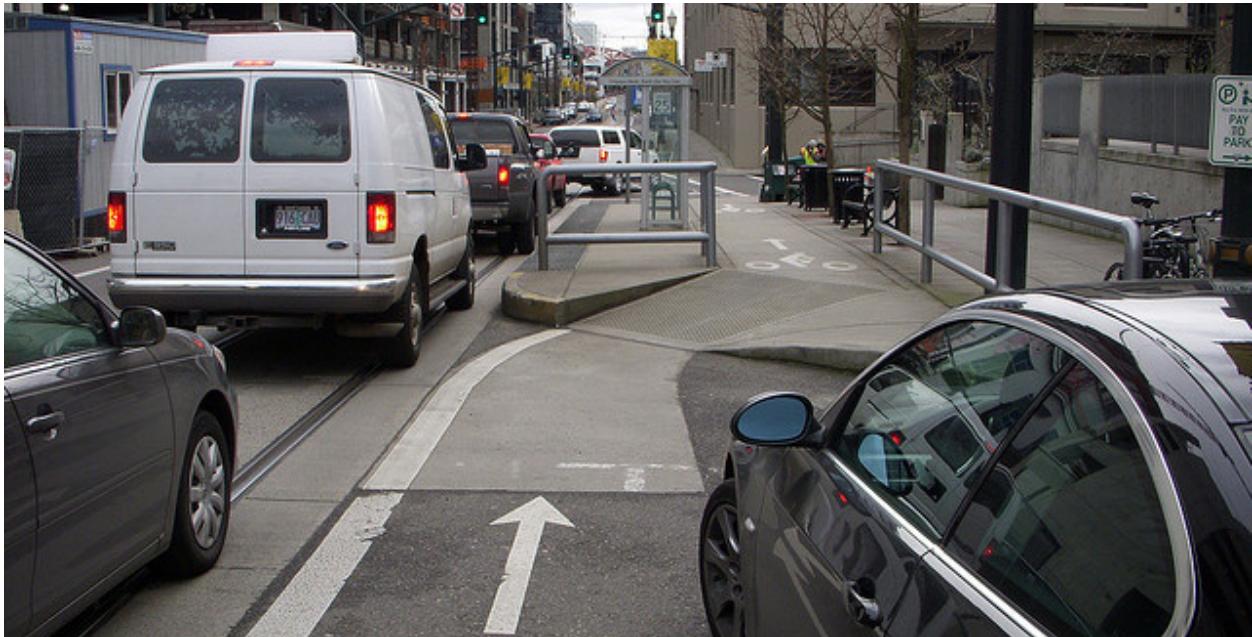
FIGURE 8.5 GRADE SEPARATED BIKE LANE APPROACHING STREETCAR STOP
