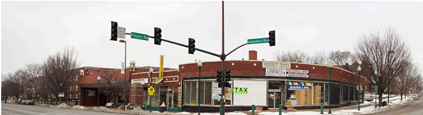
FIGURE 12.32 THE INTERSECTION OF INDEPENDENCE BOULEVARD AND PROSPECT AVENUE; VIEW FACING NORTH
