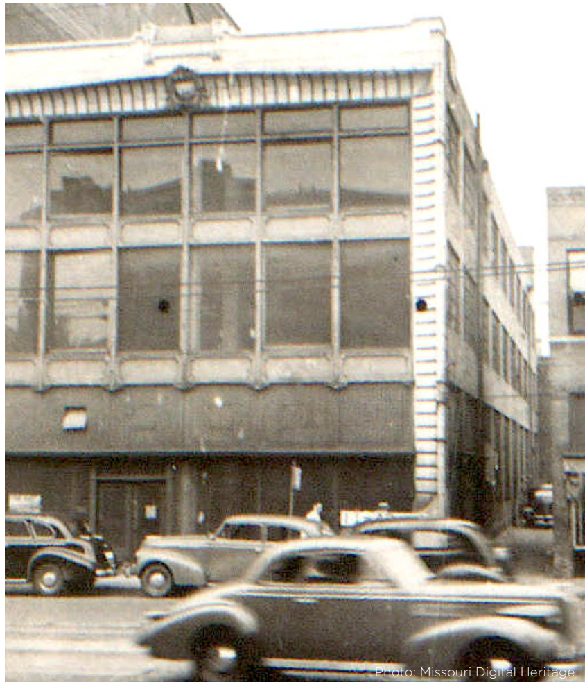
FIGURE 12.3 ABC STORAGE (1908; PREST, 1909; SMITH REA AND LOVITT 1912); 3240 MAIN STREET (FRANK JACKSON AND FREDERICK MCILVAIN, 1914), VIEW FACING WEST, 1940
