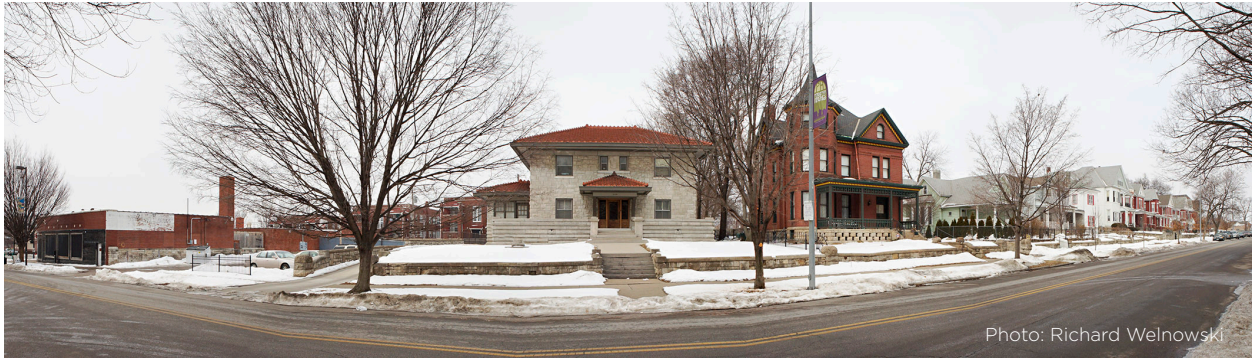
FIGURE 12.35 PENDLETON HEIGHTS WITH THE JOHN CONOVER RESIDENCE, CENTER; VIEW LOOKING NORTHWEST
