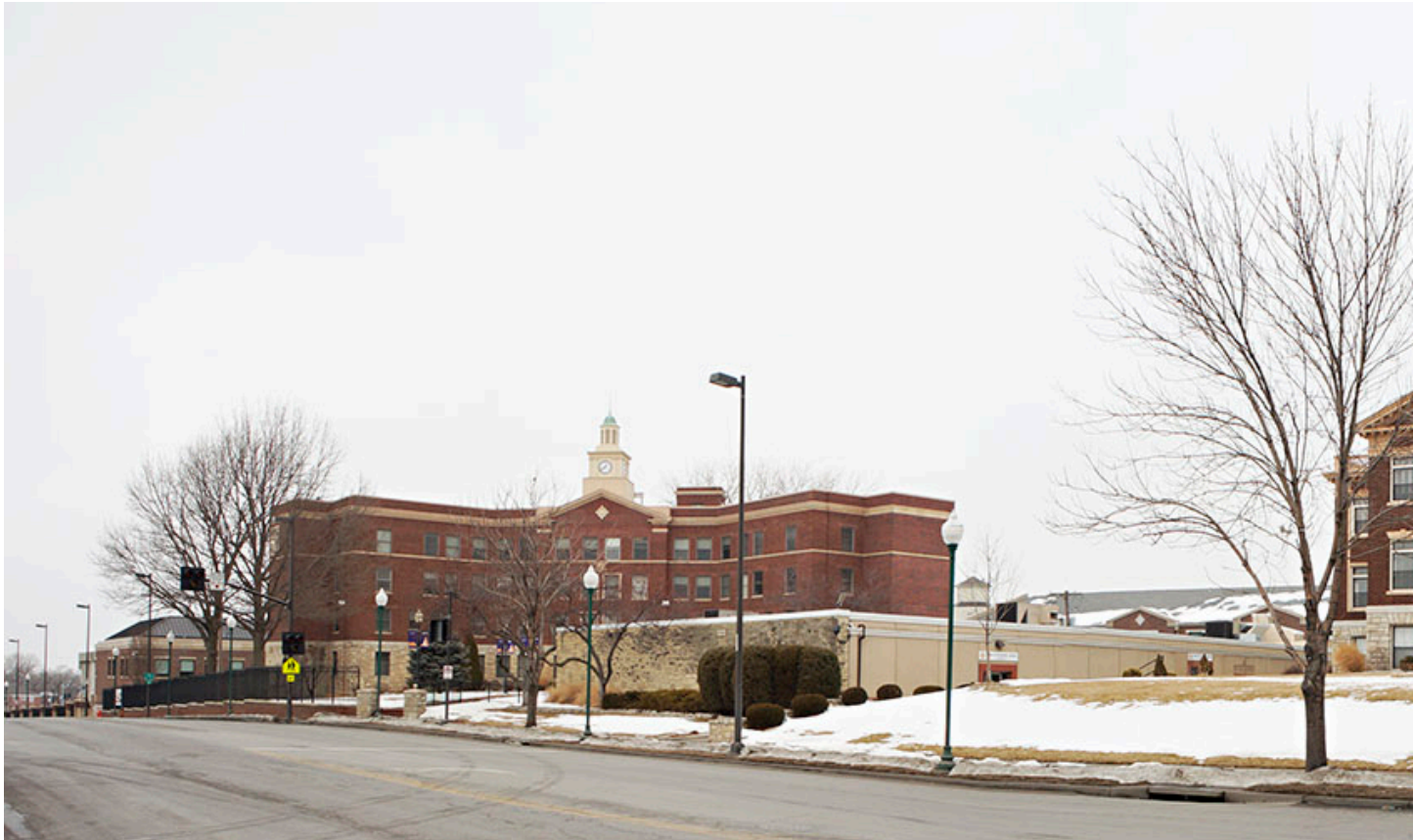
FIGURE 12.28 INDEPENDENCE BOULEVARD EAST OF THE PASEO BOULEVARD; VIEW FACING NORTHWEST. CHILDREN'S MERCY NURSES' DORMITORY (RIGHT); CHILDREN'S MERCY HOSPITAL (LEFT)
